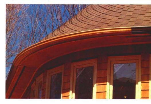
meets, and the effect (photo above) is of one continuous gutter that wraps around the house. Where the gutters joined, the connection was thoroughly coated with fiberglass. This solution wasn't entirely effective, however, and there was some leakage as the fiberglass separated from the aluminum. A liberal application of silicone sealer solved the problem.
