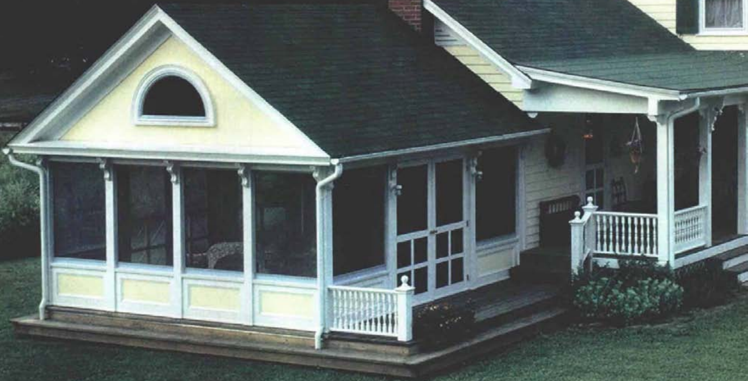
A place to kick back and relax. The screen porch the author built on his own house combines Victorian detailing with a builder's considered construction methods. In the photo below, a single pressure-treated step runs all the way around the outside of the porch as a sort of plinth.
