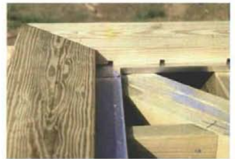
Get hip. This floor system, which is framed like a shallow hip roof, allows water to run off the porch floor. Strapped joists bring the finish floor flush with the 2x8 coping.
