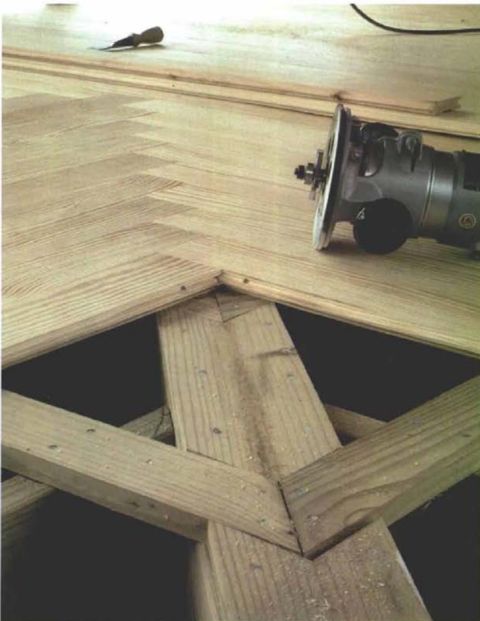
The hipped floor slopes in three directions to shed water that blows through the screens (above). Sun hitting the finished floor gives a pleasing effect. The joists are cross-strapped, and the flooring is laid on the strapping so that it runs parallel to the slope of the porch floor. A router grooved the end of each piece of flooring (below) so that it could herringbone its way down the floor's hips.
