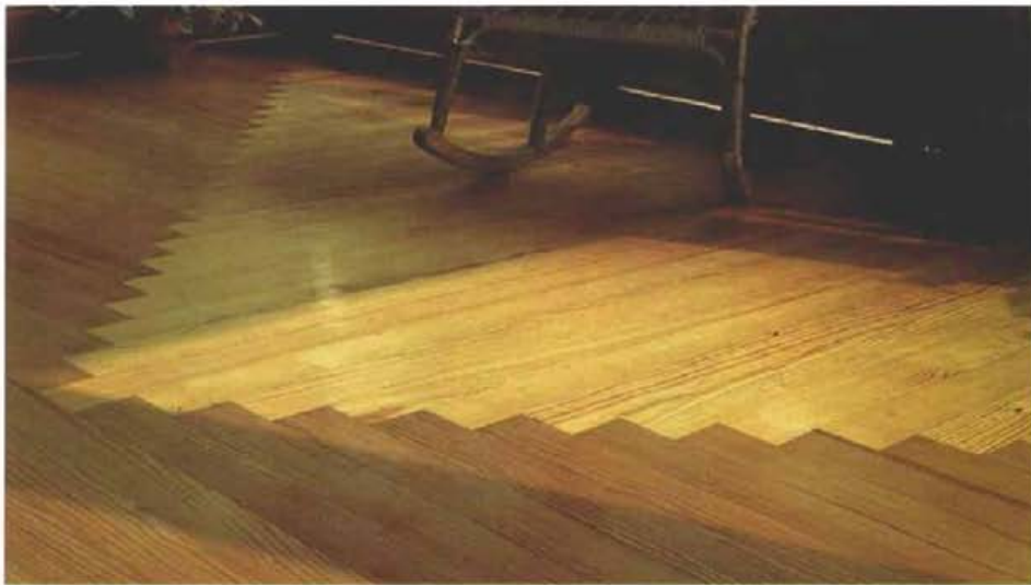
The hipped floor slopes in three directions to shed water that blows through the screens (above). Sun hitting the finished floor gives a pleasing effect. The joists are cross-strapped, and the flooring is laid on the strapping so that it runs parallel to the slope of the porch floor. A router grooved the end of each piece of flooring (below) so that it could herringbone its way down the floor's hips.
