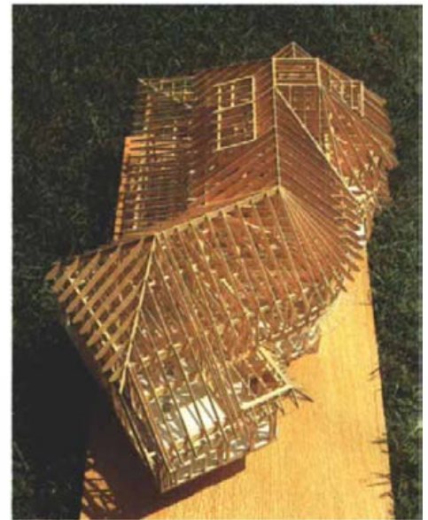
The structural model, above, shows just how complicated the roof is. The author had to deal with both an irregular plan and irregular pitches for some hip, valley and jack rafters, as well as a portion of a conical roof and dormers of several shapes. To keep on-site calculations to a minimum, he used a large developmental plan (drawing, below) that allowed angle take-offs using a sliding T-bevel, and unit measurements using a pair of dividers.
